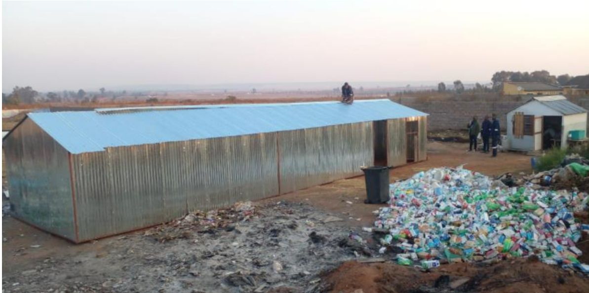
Figure 2: The building structure that Mr. Bin has built in preparation for Solar System Installation.
