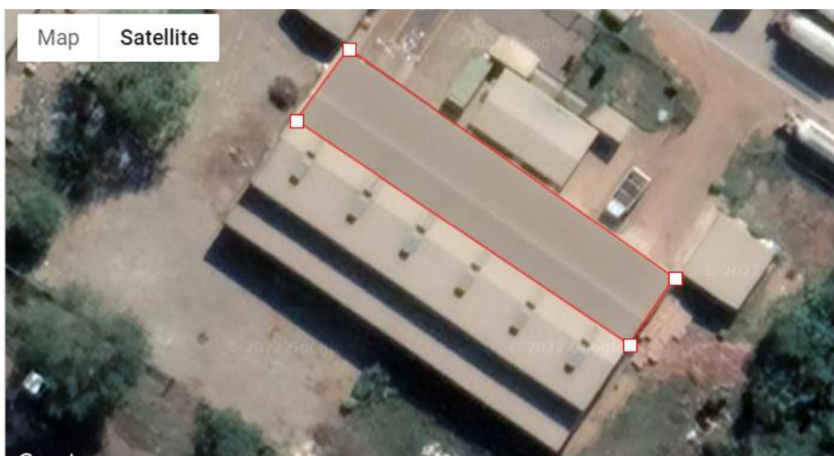
Figure 1: Eco Care Premises and their potential to generate solar energy.
